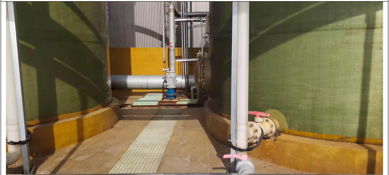
罐区收集渠及收集井
